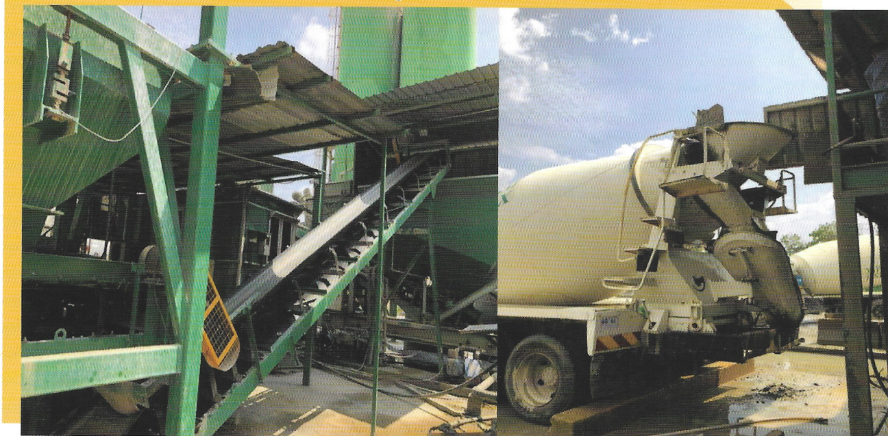
Dry Plant - Drum Mixer
